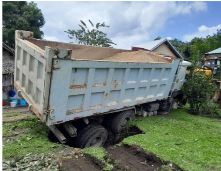
Figure 13: Truck falling in a decommissioned septic tank at the Tata School in Santo, Vanuatu
