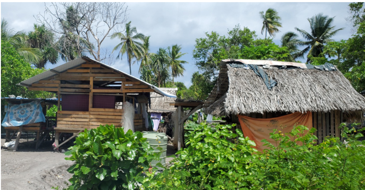
Figure 5.5 Informal construction, timber frame, closely spaced near vegetation
