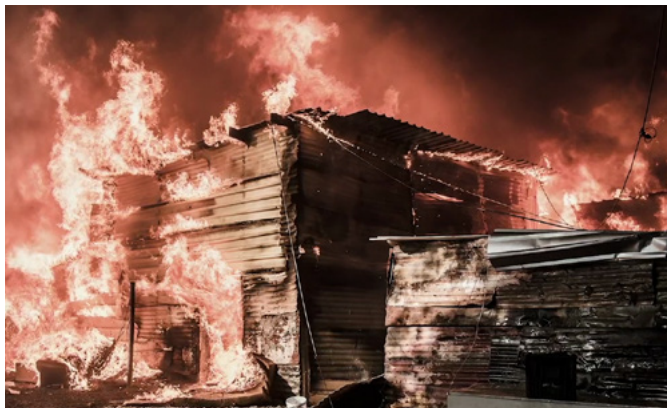
Figure 2.2 Fully involved fire of informal construction building
