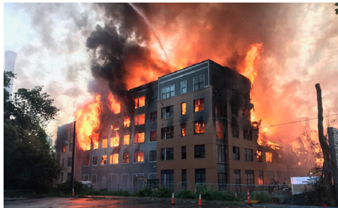
Figure 2.3 Timber frame building fire (formal construction)
