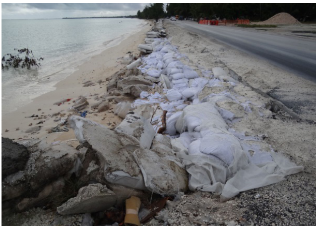
Ecological effects of coastal structures. Two examples of adverse effects of engineered coastal structures are: at left, synthetic materials released when a structure breaks down; and at right, the trapping of debris Source: The authors.
