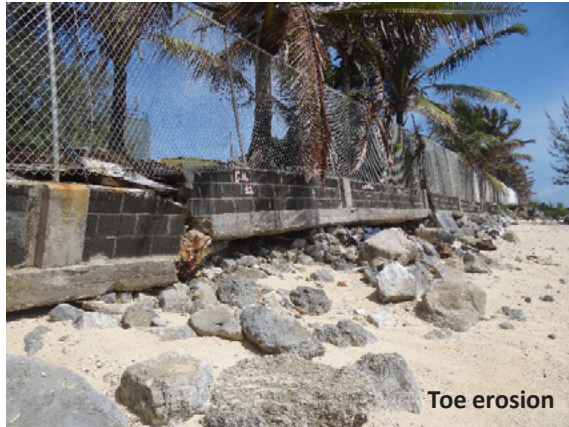
Figure 16: Examples of Typical Failure Mechanisms in Coastal Protection Works on Pacific Islands
