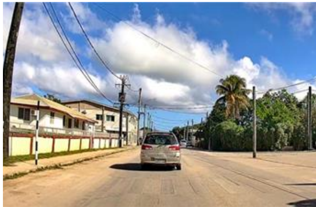
Lack of Visible Zebra Crossing, Signages, etc.
