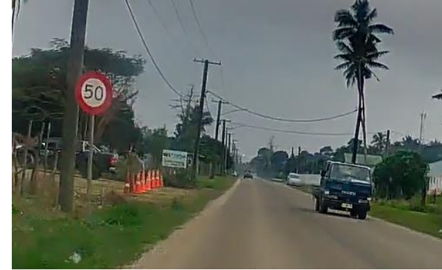
High Operating Speeds (40–60 km/h) in Town Center and Near Schools
