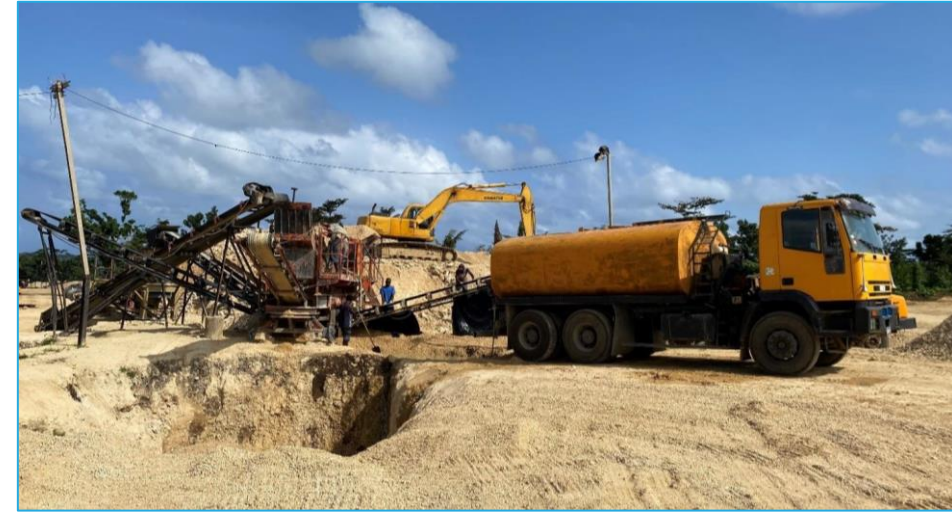
Washing of crushed limestone aggregate, Efate, Vanuatu (photo: Paul Rogers, 2023)
