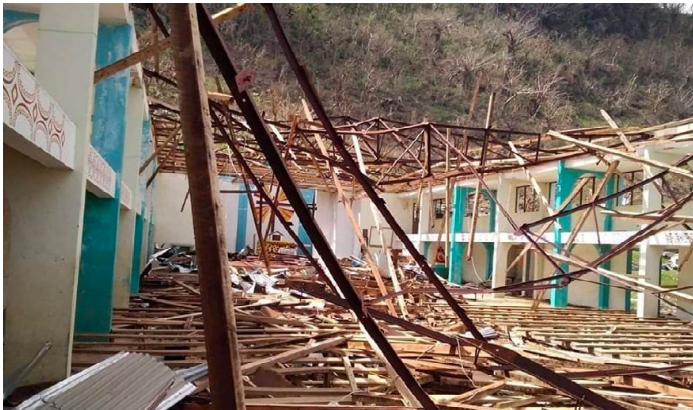
Melsisi Catholic Church Vanuatu following the destruction of Tropical Cyclone Harold in April 2020. Source: Naparau Jelson Nishai
