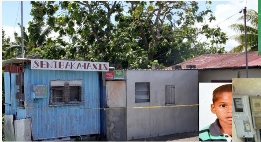
The electrical wire in which, Tomasi Melb Kaivu, 6 was electrocuted at Lami village on Friday afternoon. PHOTO: Arieta Vakasukawaqa.
