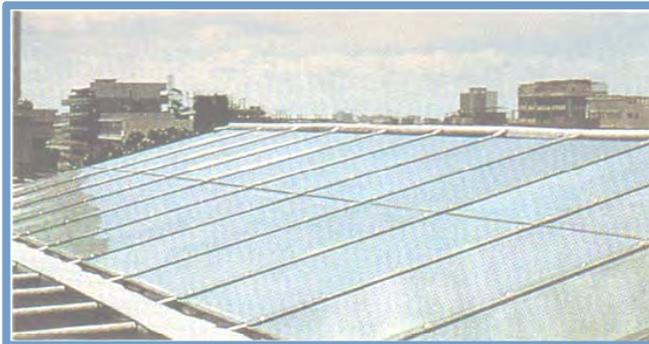
*Flat-Plate hydronic collectors* have a delivery temperature typically between 110 F and 160 F (43.3 C - 71.1 C). They are primarily appropriate for domestic water heating. They function using a thermosyphon, where natural circulation takes place based on the density of hot or cold water. Efficiency is typically around 30% - 35%.
